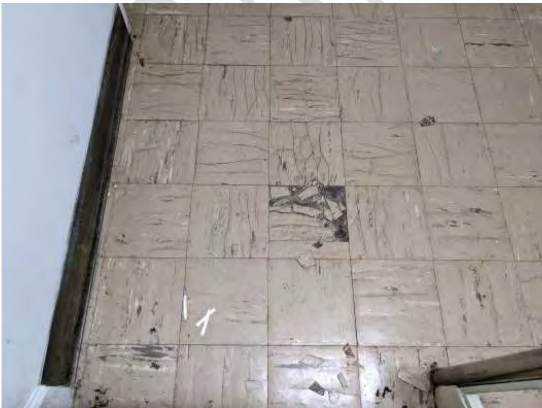
Photograph 8: Asbestos tiles
