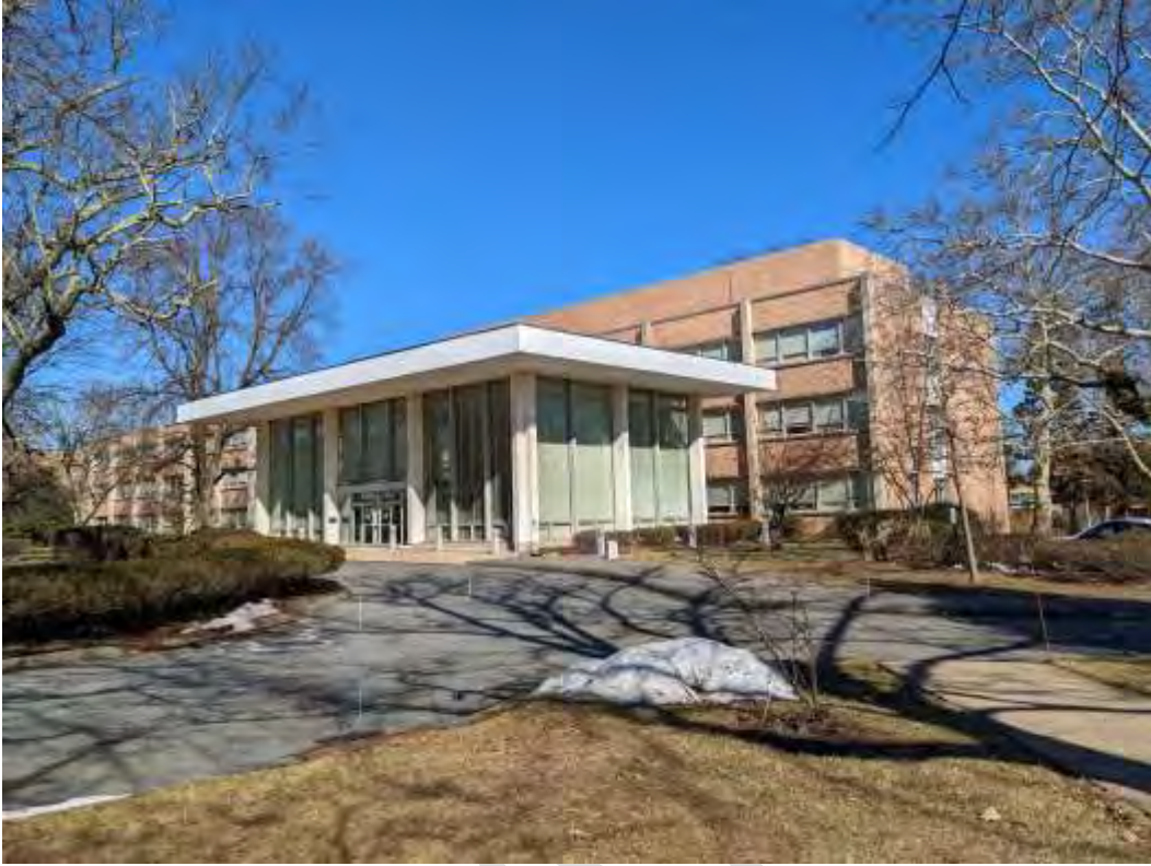
Photograph 3: Main Entrance Lobby
