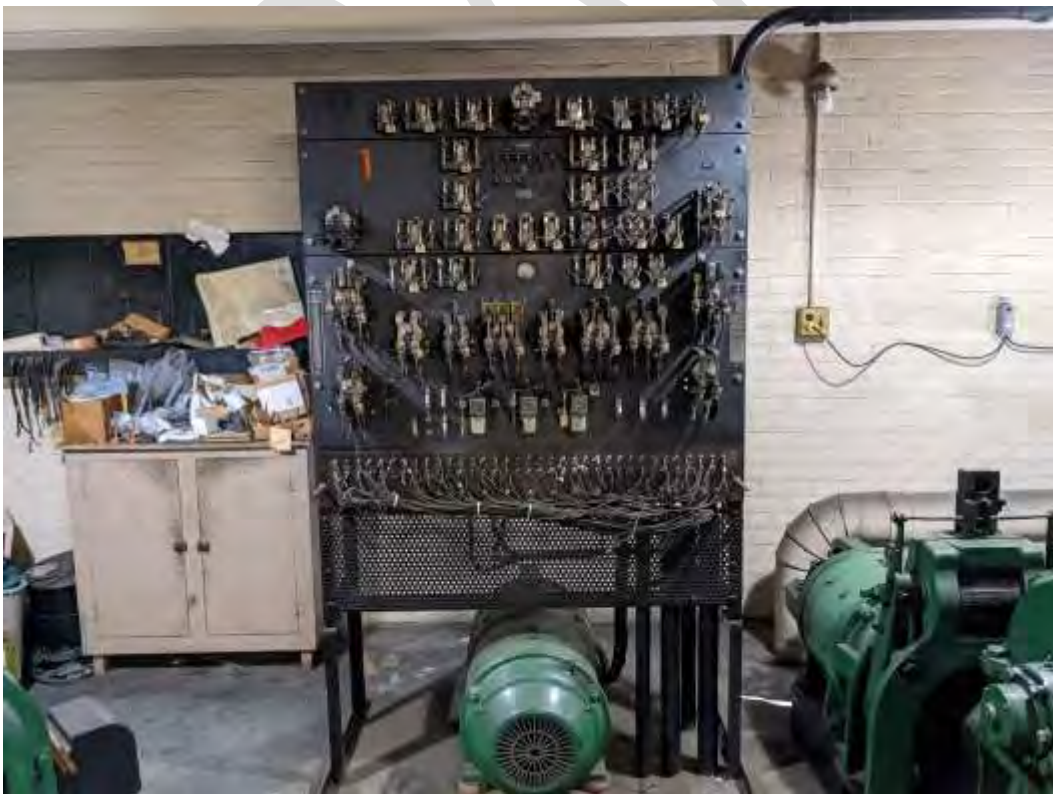
Photograph 21: Original elevator infrastructure
